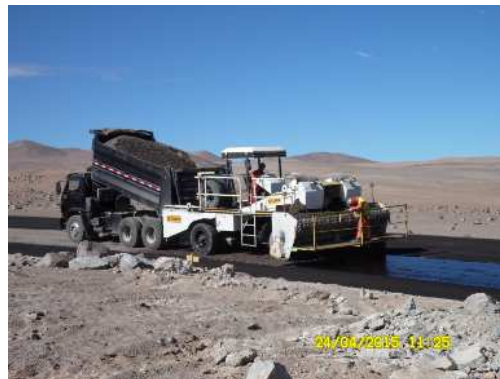
Fig. 4. Asphalt work on the access road to Armazones
