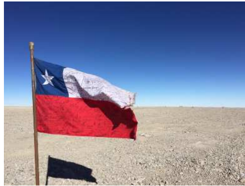
Fig. 3. The top platform at Armazones after flattening by the company ICAFAL whose workers proudly signed the Chilean flag seen in the foreground at completion of the work.
